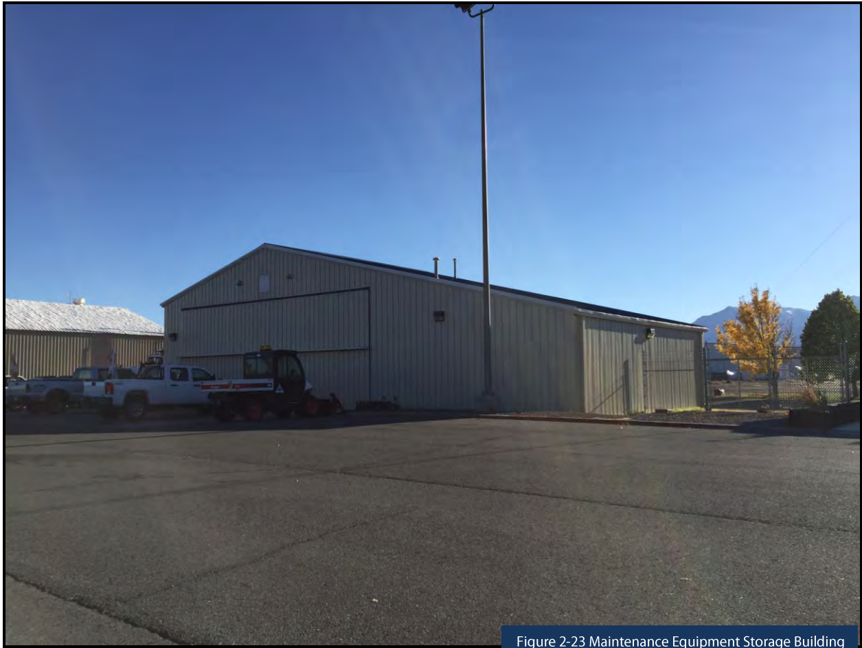
Figure 2-23 Maintenance Equipment Storage Building
