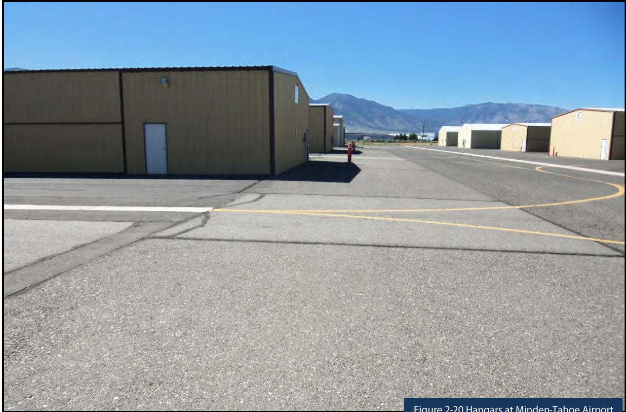
Figure 2-20 Hangars at Minden-Tahoe Airport
